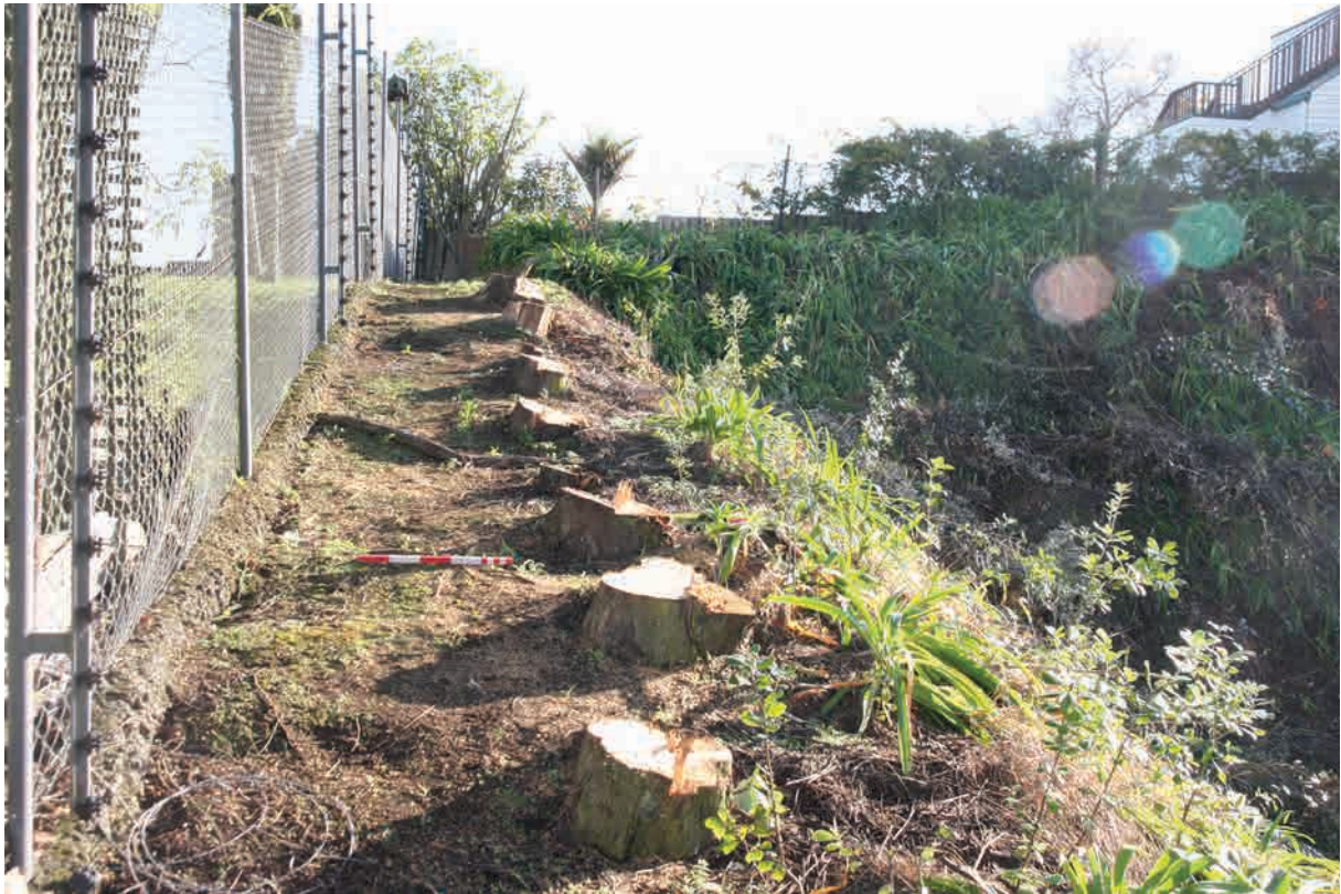
Figure 15. Top of the batter in the Lot 1 DP 194641 in 2019, showing recently cleared conifers.
